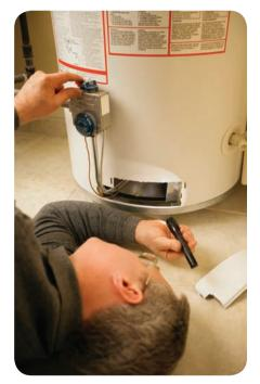
▲ Gas-fuelled water heaters and boilers should be checked regularly. Every year, hundreds of people are killed by carbon monoxide from faulty burners.
