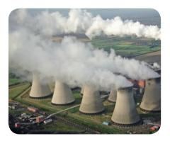
Most of the rest is burned for heat, in factories, homes, and power stations, as above. In a power station, the heat is used to turn water to steam, to drive turbines.
