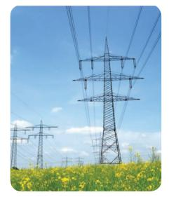
▲ Electricity cables: aluminium (light) with a steel core (strong).
