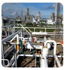
▲ Ammonia plants are often built close to oil refineries, to make use of the hydrogen from cracking.
